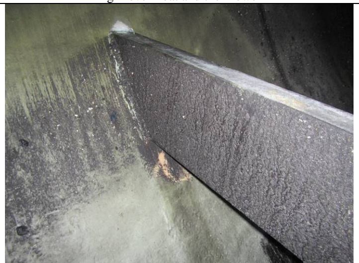
Fire tube supports welded to shell – no corrosion or damaged coating
