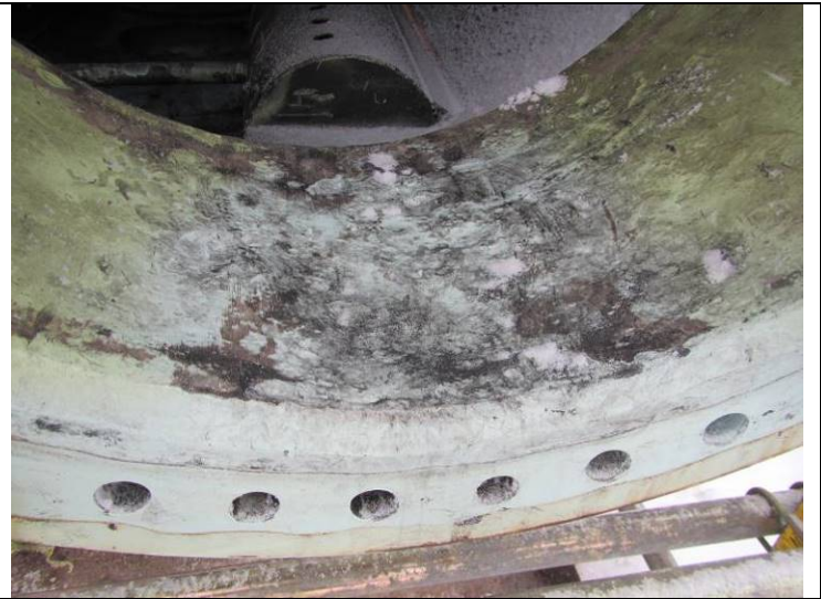
Previous corrosion on fire tube access
