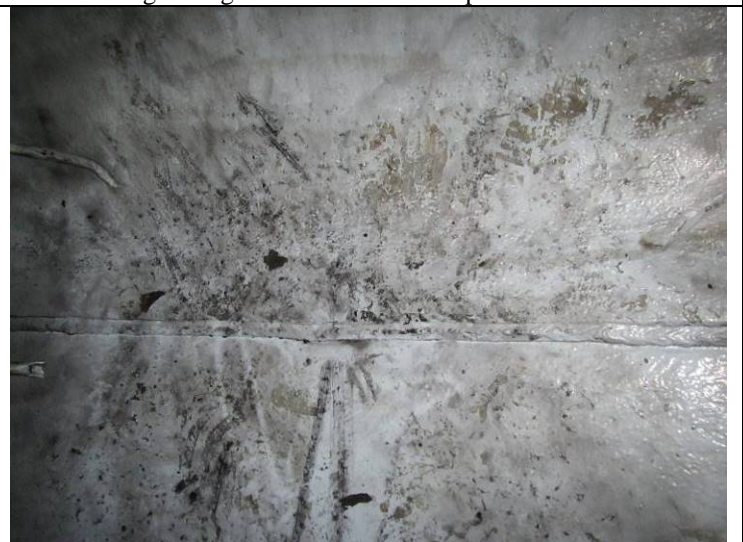
North head to shell weld
