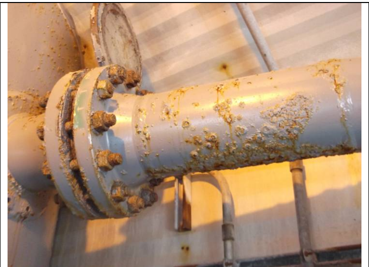
External corrosion
